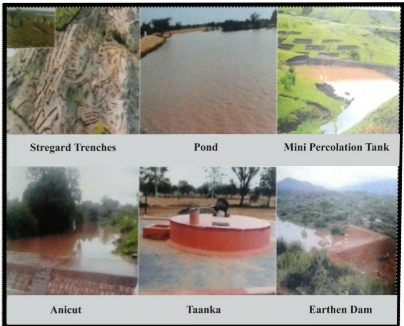
Fig. 8.15 : Various forms of Water Conservation
